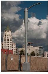
Ericsson has created integrated cellular technology that incorporates 4G LTE network radios in the form of street lights called small cells. By supplementing existing cellular towers, the Philips' Smartpole Street Lighting uses existing towers with small cells to provide wider mobile broadband coverage while boosting the capacity of wireless providers. Los Angeles is the first city in the world to acquire this technology.
